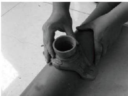
4. Install the Mechanical Tee in the hole.
