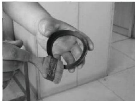
2. Spread lubricant on gasket ring.
